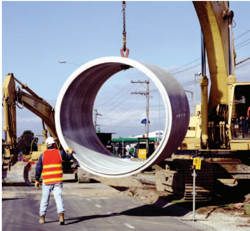
Replacing a stormwater pipe. Photo: Tracey Nicholls, CSIRO.
